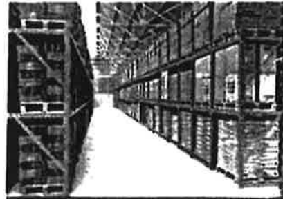
Pallet racking made from Dexion slotted angle
